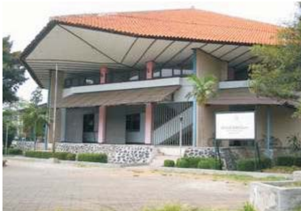
Fig.4, Multiple use building in Rusun Klender, Jakarta Source: Study of Debt Swap Scheme Policy for Housing Development Budget, 2007
